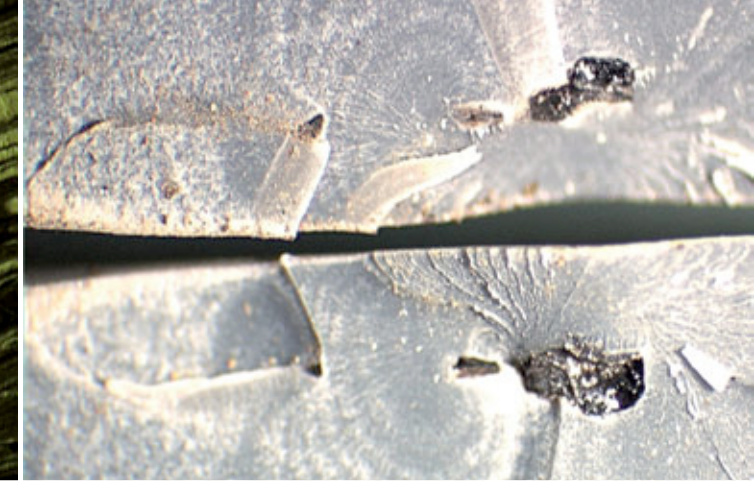
Pipe fracture caused by impurities
